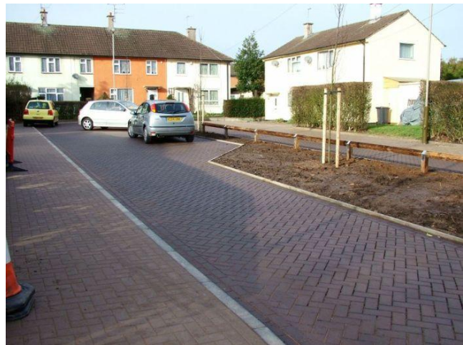
Figure: Implementation of Abbey Lane Sustainable Urban Drainage System in Leicester
