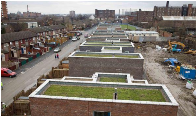
Figure: Manchester is adapting to climate change is through its work on green roofs. (Source: Wild About Manchester, Green Roof Studies)
