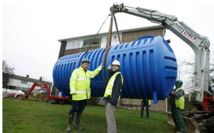
Figure: Installing rainwater harvesting tank beside block of flats (Source: Preston Water Efficiency Initiative, Final Report, March 2009)
