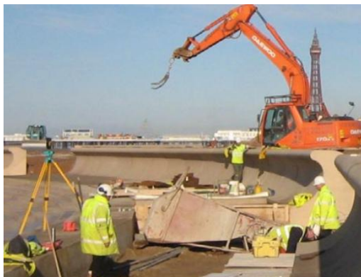
Figure: Reconstruction and improvement of damaged sea defences. (Source: ReBlackpool Annual Report, 2008)
