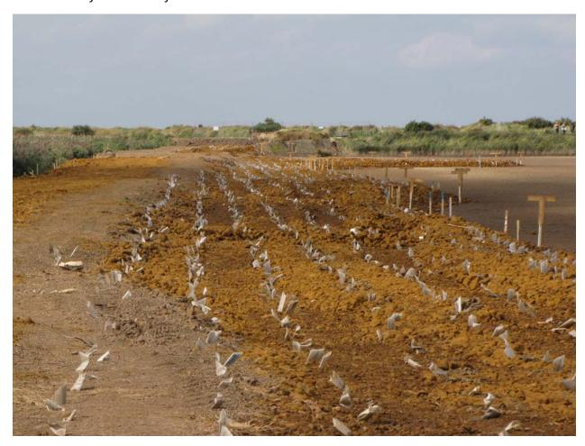
The excavated lime-treated material was then transported by dumper truck along the haul road and placed onto the Parrinder bank. To provide the stability required, the sea bank was built up in layers wrapped with geotextiles and compacted.
