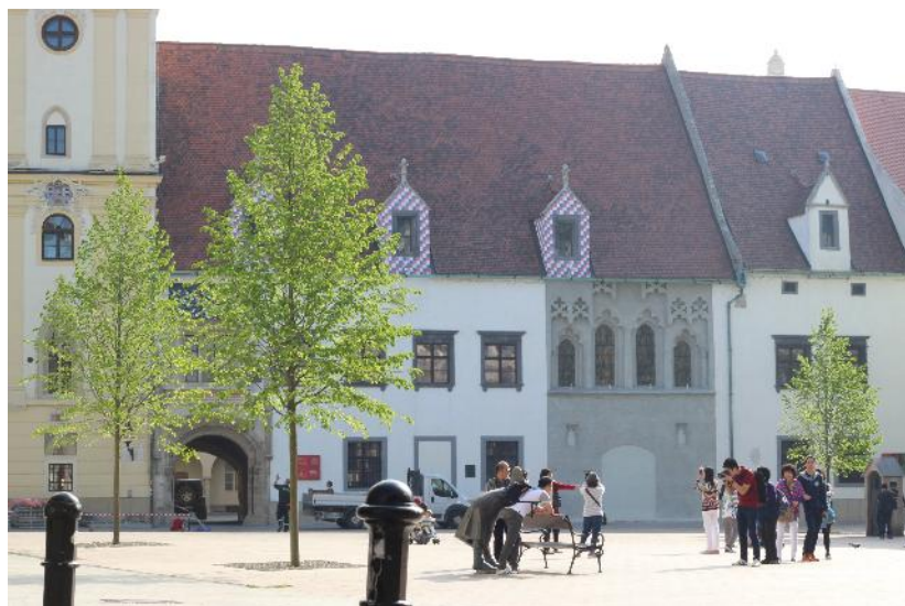
Fig. 10: Planting new trees and planting trees in previously only paved squares in the Old town. (Photo source: Office of the Chief Architect, City of Bratislava)
