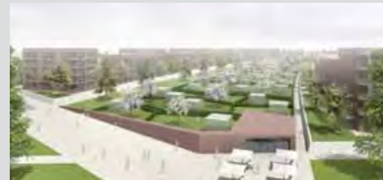
10 Roofed section of the A7 motorway, Altona
