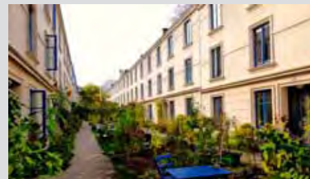
46 Green courtyard, Falkenried Terraces
