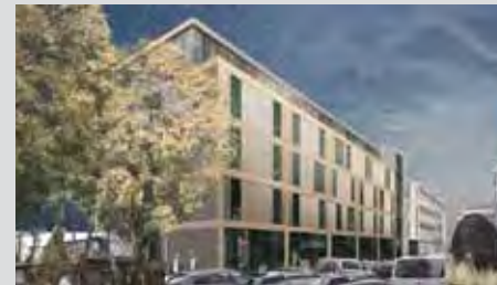
61 Eifflerwerk, hub for networks and innovative start-ups, St. Pauli
