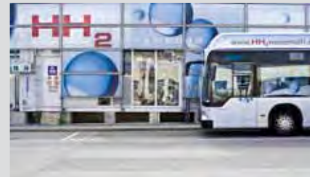
53 Hydrogen filling station, HafenCity
