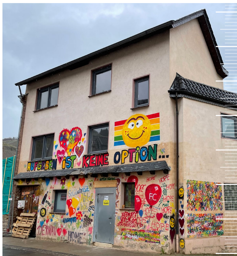
'Giving up is not an option' – painted façade of a house in Dernau, Germany, April 2022. Photo: Michael Szönyi
