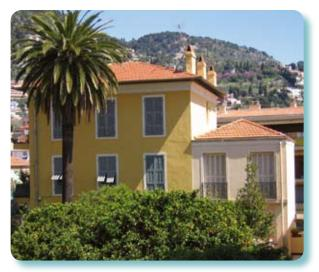
**Figure 15:** Shutters are used widely in warmer climates to provide shade. These shutters are slatted and can tilt at the base so that ventilation can still be provided via opened windows during the day.
