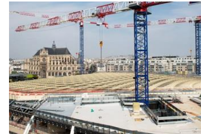
Renovation of Les Halles district
