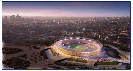
The London Olympic Stadium is said to be the most sustainable ever built. It has been made from materials 75 percent lighter than steel, the most common material used to build other stadiums. Lowcarbon concrete was used in its construction, which contains 40 percent less carbon than usual. Steel and
