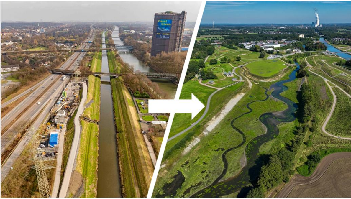
Figure 2: In areas where there is sufficient space, the canalised river can be transformed into a free-flowing Emscher. The Emscher in Oberhausen (left) and the Emscher in Castrop-Rauxel (right) demonstrate the potential of this approach. Image Credit: EGLV.
