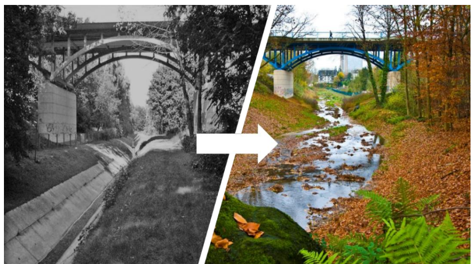
Figure 4: Revitalised stream (Borbecker Mühlenbach) as an example for the successful restoration of the smaller tributaries in the Emscher catchment area. Image Credit: EGLV.
