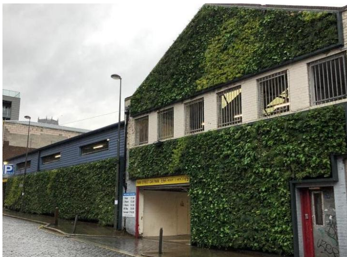
Figure 3: Green wall implemented at Parr Street, Liverpool. Source: URBAN GreenUP . Image Credit: Julite Staples.
