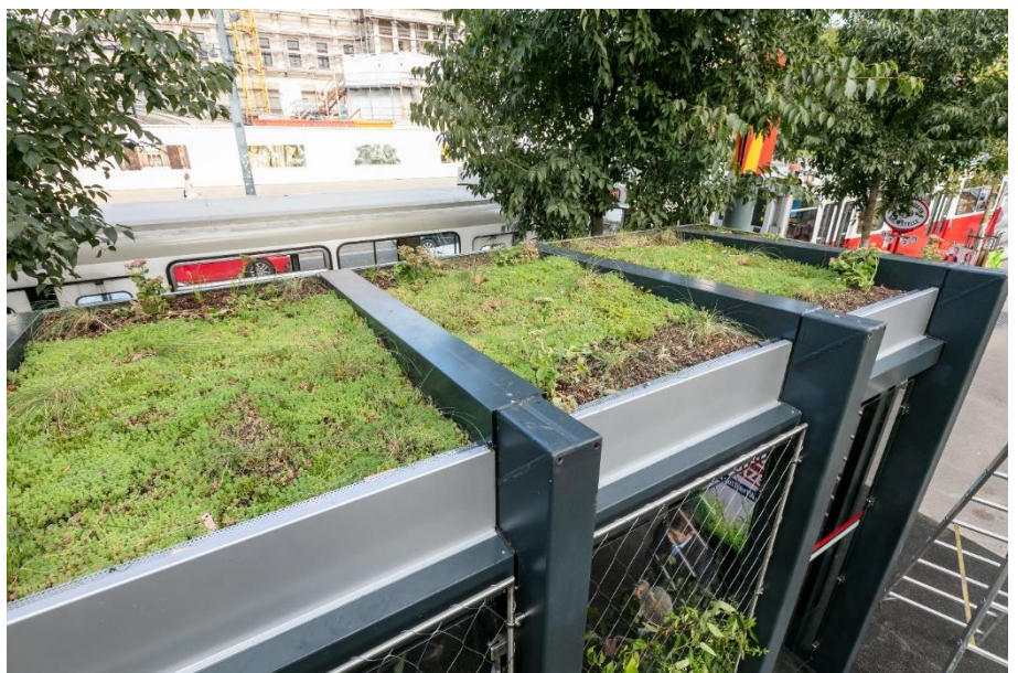
Figure 1: A completed climate-adapted bus stop with a green, vibrant roof, also supporting biodiversity. Image Credit: Wiener Linien.
