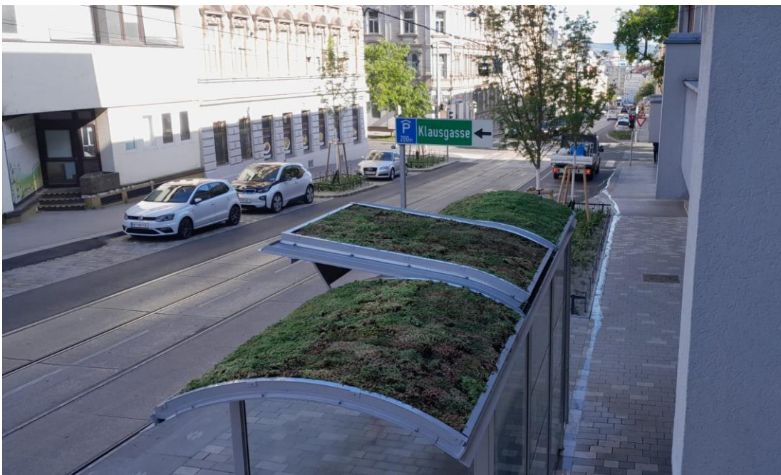
Figure 3: A more practical type of climate-adapted bus stop with sedum mats. Image Credit: Wiener Linien.
