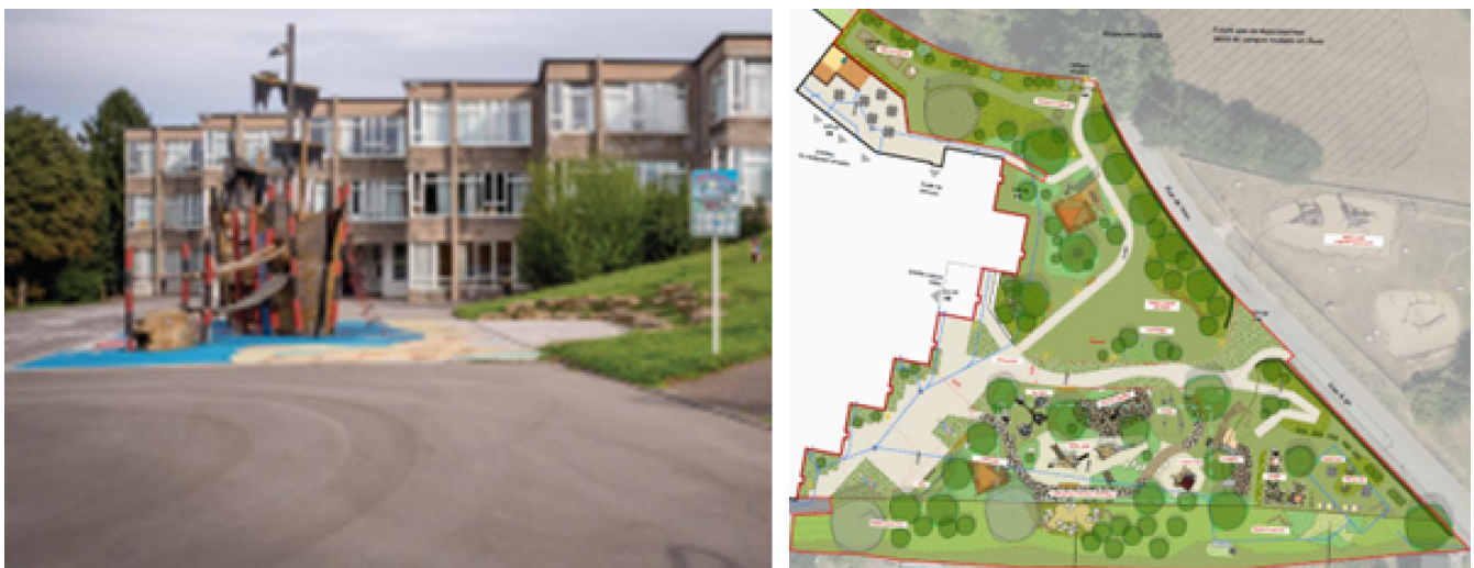
Figure 3: School grounds before (left) and after (right). Image Credit: Ville de Differdange.
