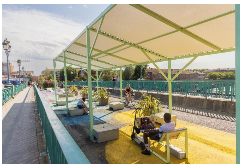
Figure 2: Shading structures at mbrière pont Saint-Pierre (Image Credit: P. Nin)
