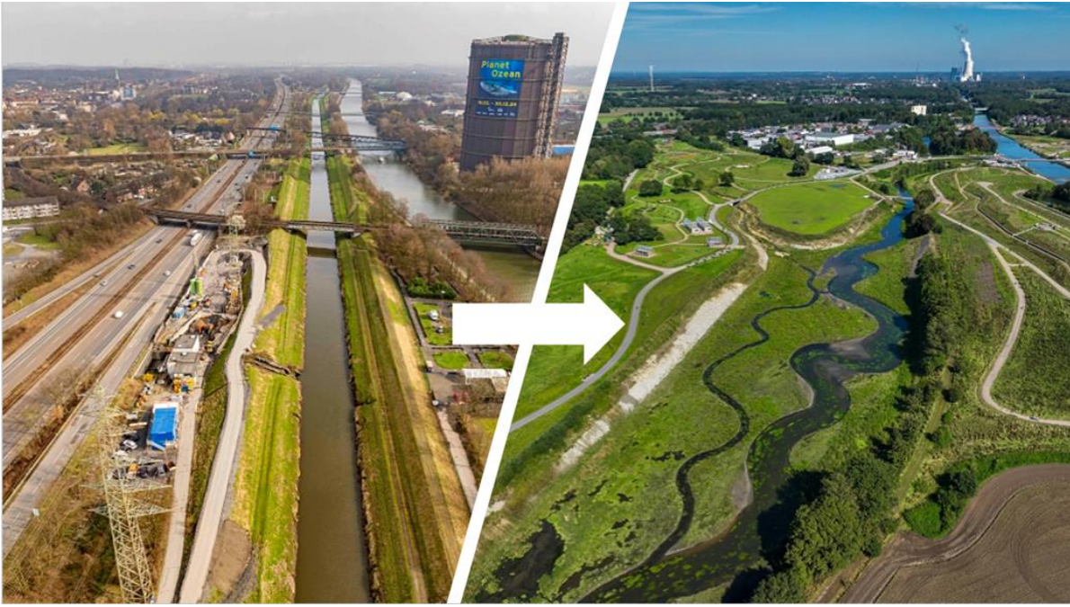
Figure 2: In areas where there is sufficient space, the canalised river can be transformed into a free-flowing Emscher. The Emscher in Oberhausen (left) and the Emscher in Castrop-Rauxel (right) demonstrate the potential of this approach. Image Credit: EGLV.
