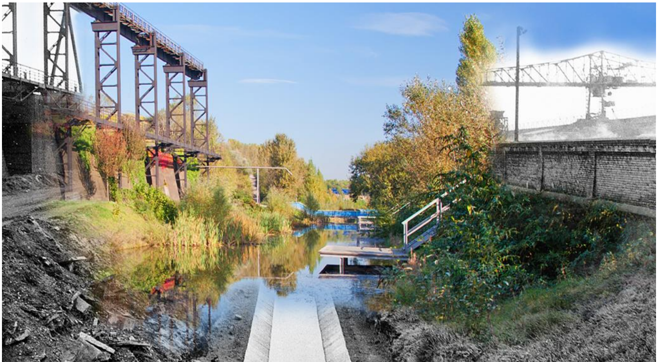
Figure 3: Visualisation from a grey, canalised sewer system to a blue-green infrastructure with revitalised streams in the Landscape Park in Duisburg. Image Credit: EGLV.
