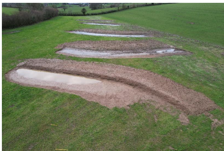
Figure 1: Scrapes and Sediment Traps at Snowdon Hill Farm. Image Credit: Iorwerth Watkins, Westcountry Rivers Trust
