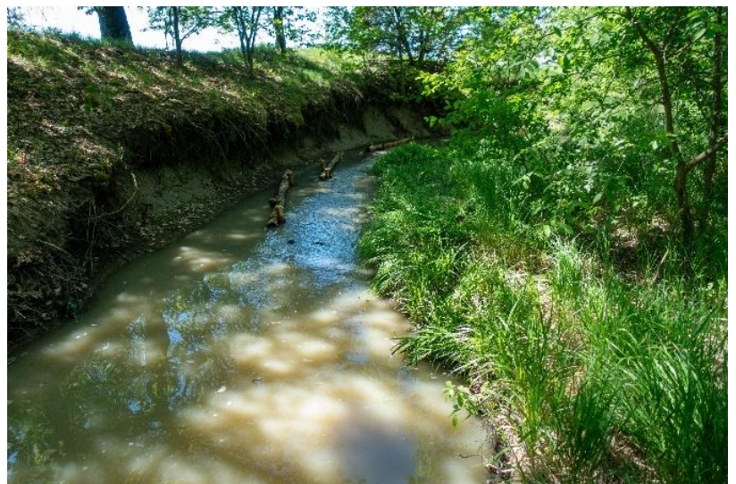
Figure 5: Wooden deflectors were installed in the eroded channel of the Myllyoja stream to prevent further erosion and to create additional flowing water habitats. Image Credit: Omar Badawieh.
