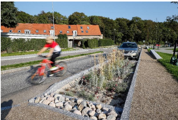
Figure 6: Roadside infiltration beds to slow down speeding cars and provide new green elements. Credit: City of Aarhus
