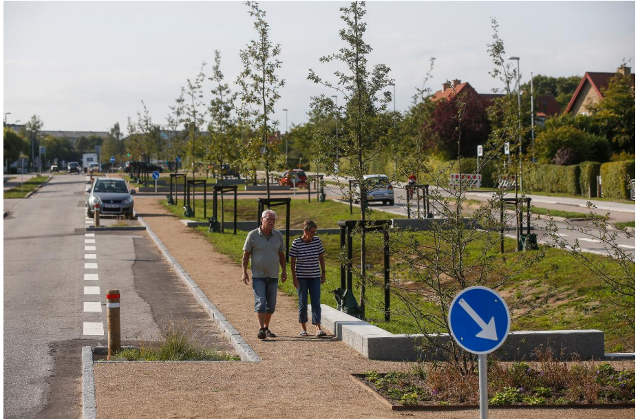
Figure 5: Green depressions at the middle of the road to make space for stormwater. Credit: City of Aarhus.
