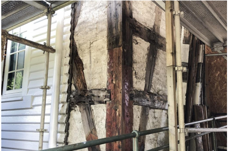
Figure 2: An uncovered corner of Mandal church showing how the cladding was connected directly to the wooden construction. Fungi and rot had damaged the structure. Image Credit: Tanja Røskar/Multiconsult.
