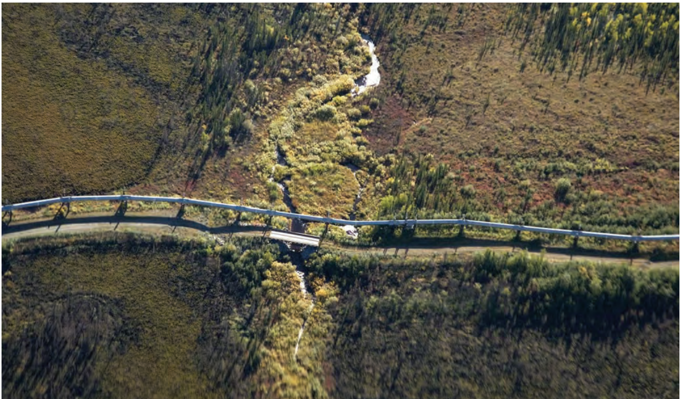
Fees collected for pipeline rights-of-way can be a significant source of income for urban protected areas. US Fish and Wildlife Service.
