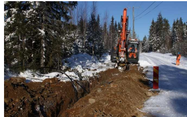
Replacing overhead lines with underground cables in Finland
