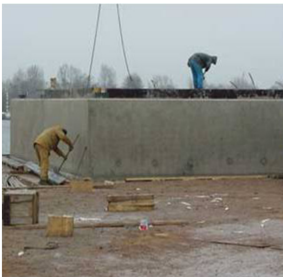
Prefabrication of concrete hulls on site.
