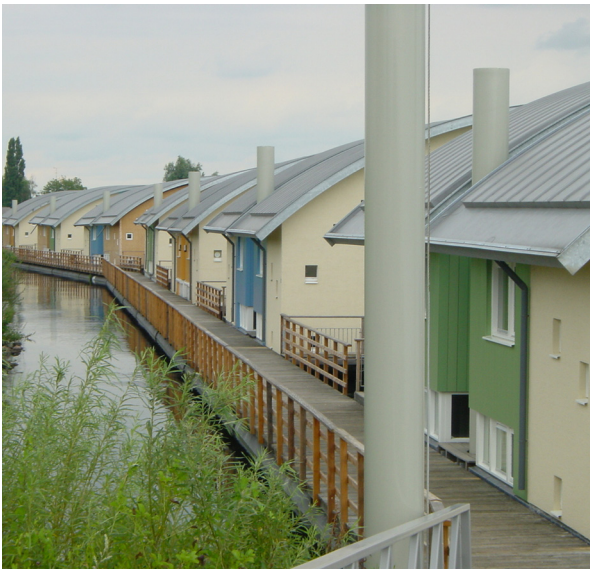
Floating homes seen from access road, July 2005.
