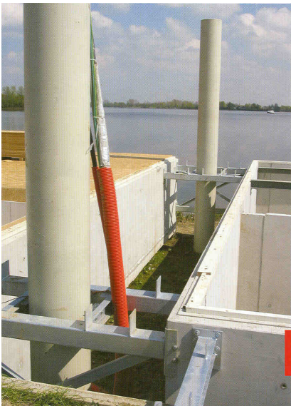
Flexible facility connections between two houses, before connection to the house.
