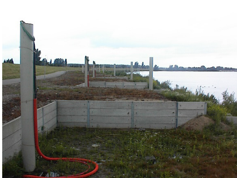
Flexible facility connections between two houses, before connection to the house.
