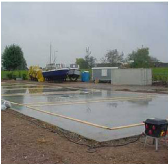
Prefabrication of concrete hulls on site.
