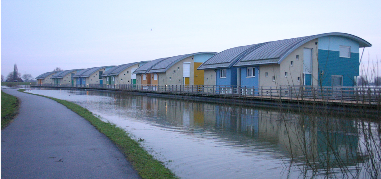
Floating homes seen from the dyke, January 2011.
