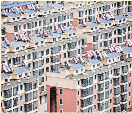
Solar water heaters on newly built apartment blocks in Hunchun, China © UN-Habitat/Alessandro Scotti
