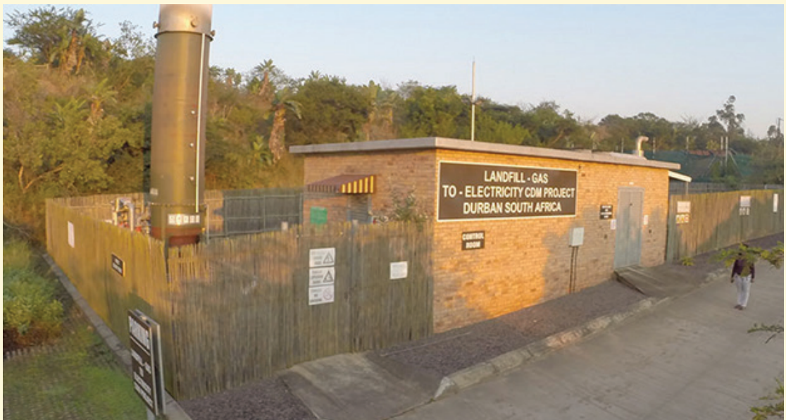
Durban landfill gas to electricity project © Fountain Green Energy
