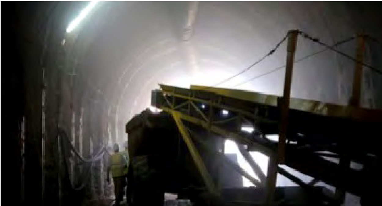
The tunnel from inside © [Di-Ve]
