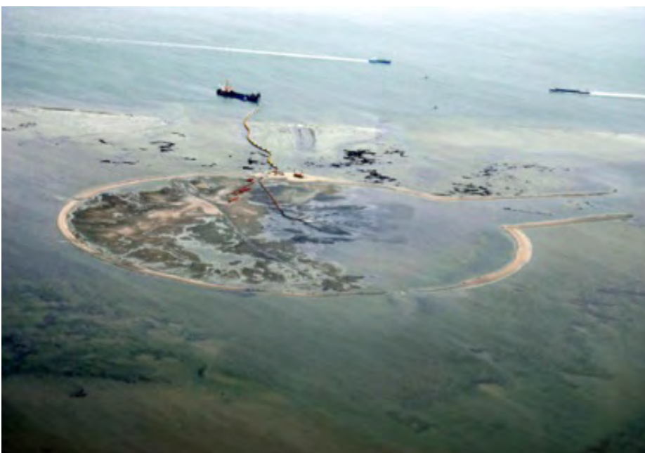
Construction of the pilot sand nourishment at the Galgeplaat
