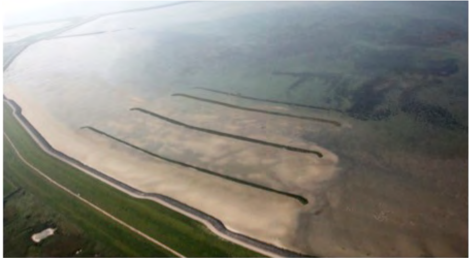
Hanging beach test site at Schelphoek
