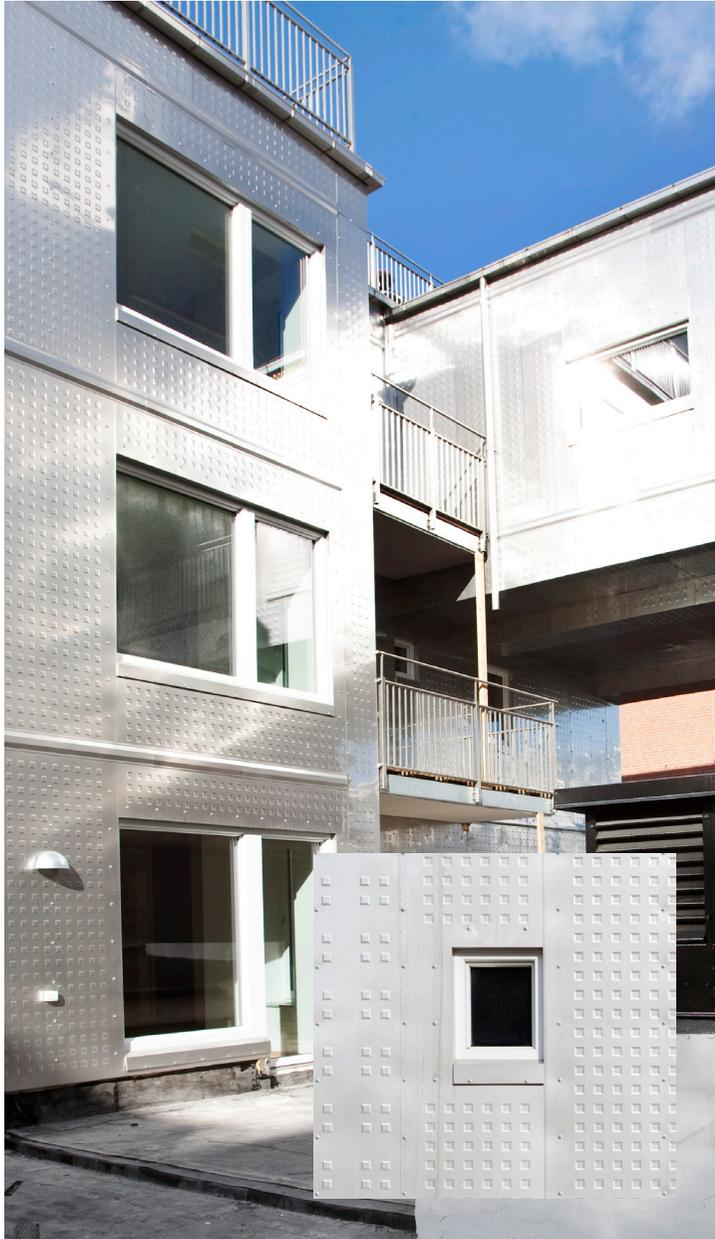
*Photo to the left: The façade is clad with steel, which glitters in the sun.*
