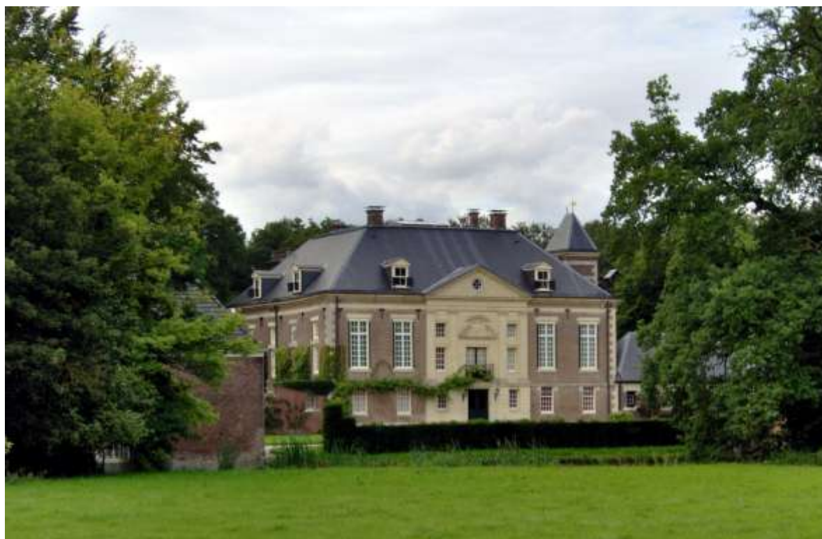
Figure 28: One of the estates: House of Diepenheim (Source: Tubantia)
