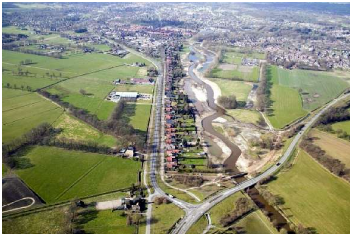
Figure 39: Veldkamp work in progress (Source: Photo Holland)
