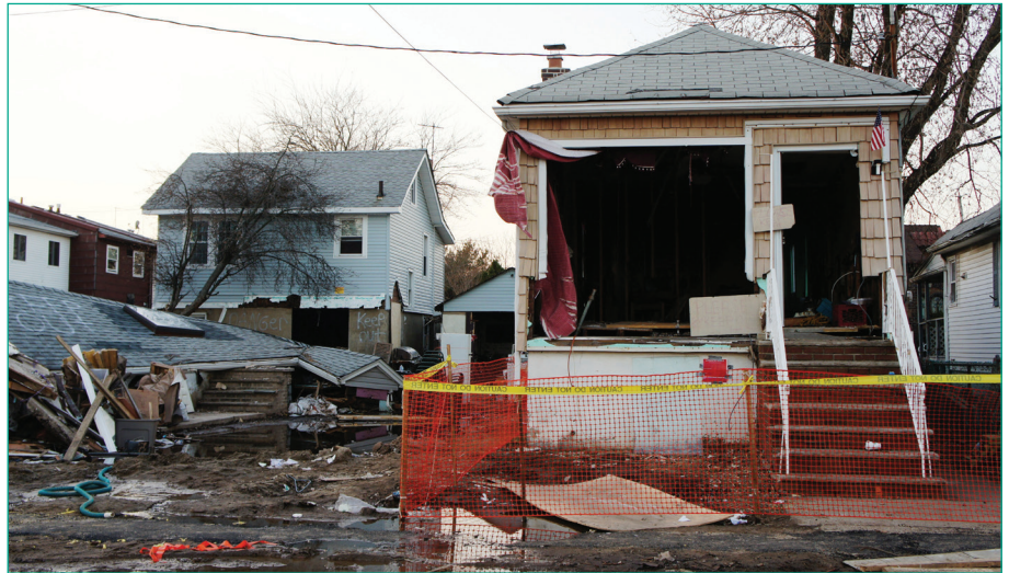
Figure 3: Damaged homes in New York City as a result of Hurricane Sandy, November 2012. Photo by Somayya Ali Ibrahim.
