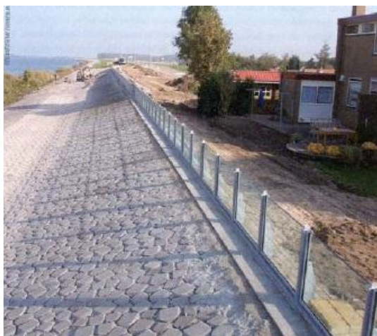
Glass overtopping walls as reinforced flood protection.
