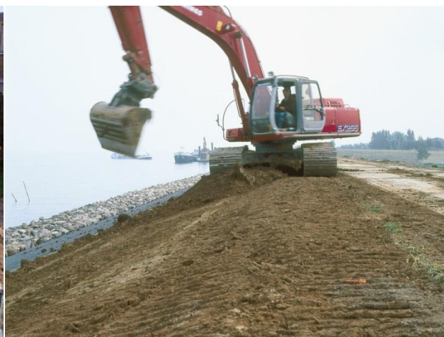
Reinforcing a dyke in Andijk, the Netherlands.
