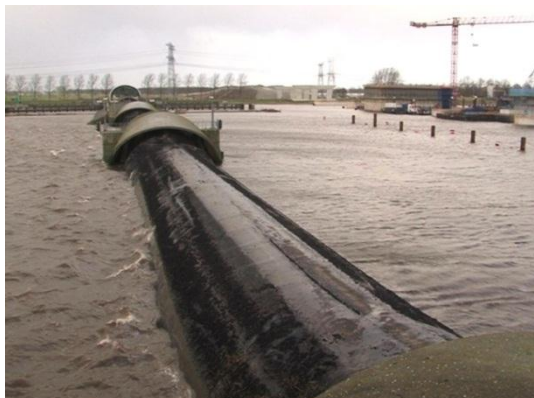
Bladder dam in the river IJssel in Kampen the Netherlands. Source: RTVOost.nl
