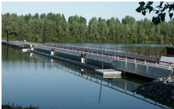
Floating road near Den Bosch, the Netherlands. Source: Dutch Ministry of Infrastructure and the Environment.
