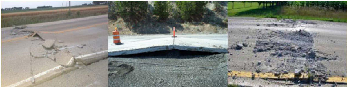
Figure 5.4 Damage to road surfaces due to weather influences (Source: Matulla & Namyslo, 2014a).
