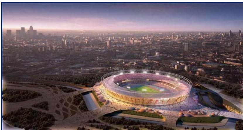
The London Olympic Stadium is said to be the most sustainable ever built. It has been made from materials 75 percent lighter than steel, the most common material used to build other stadiums. Low-carbon concrete was used in its construction, which contains 40 percent less carbon than usual. Steel and
